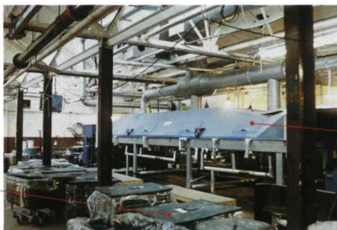
Figure 4: A factory using a combination of local exhaust ventilation and dilution ventilation to control airborne contaminants
